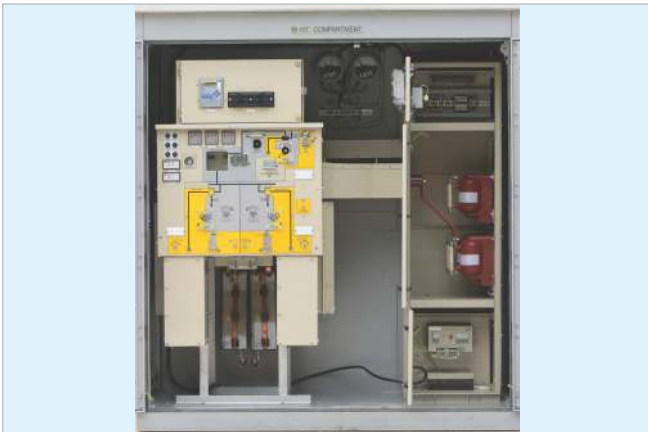
Figure 3.3: MV compartment
