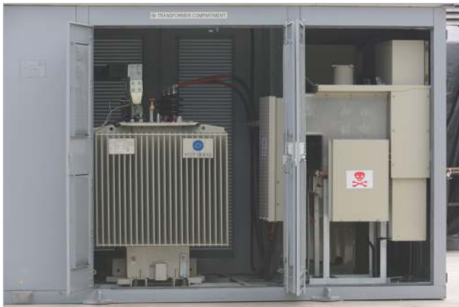
Figure 3.4: Transformer Compartment
