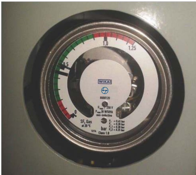
Figure 3.7.1: Gas Pressure Indicator
