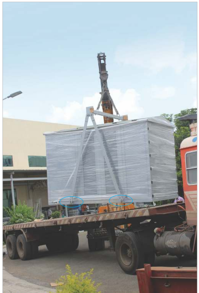
Figure 4.1.2.2: Lifting Method Of CSS
